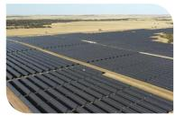
Proceeds from Vena Energy's green bond programme have been used to build out renewable energy capacity across Asia and Australia. This includes the Tailem Bend 2, a combined solar and battery energy storage system (BESS) in South Australia. The project, with 159MW capacity (118MW of solar and 41MW of battery storage), will power 35,000 homes annually and reduce greenhouse gas emissions by over 207,000 tonnes of  $CO_2e$ .
